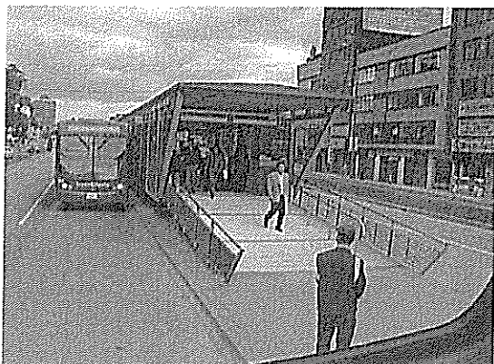
Figure 10: entrance of Transmilenio station providing access to mobility-impaired passengers
