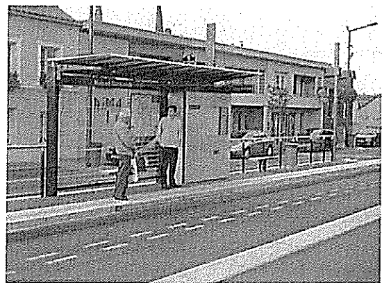
Figure 5: TEOR stop and exclusive lane in the centre of the road
