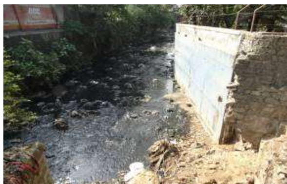
Photo 1: Nallah (Drain) Near Dahisar
