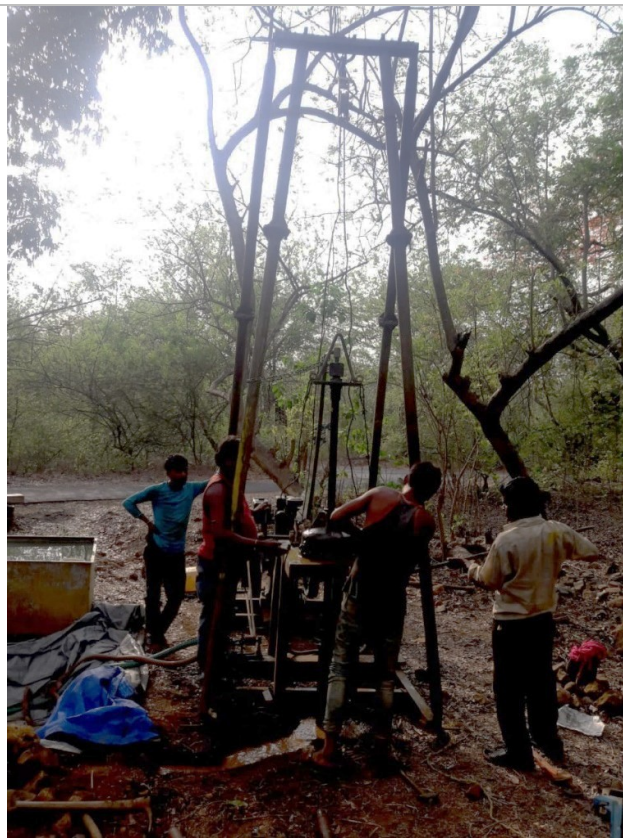
Bore Hole No. 3
