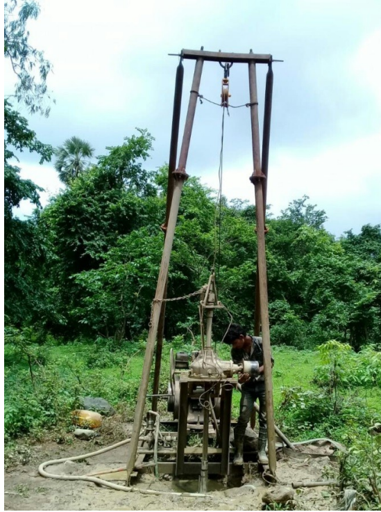
Bore Hole No. 2
