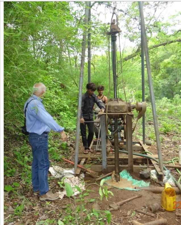
Bore Hole No. 7
