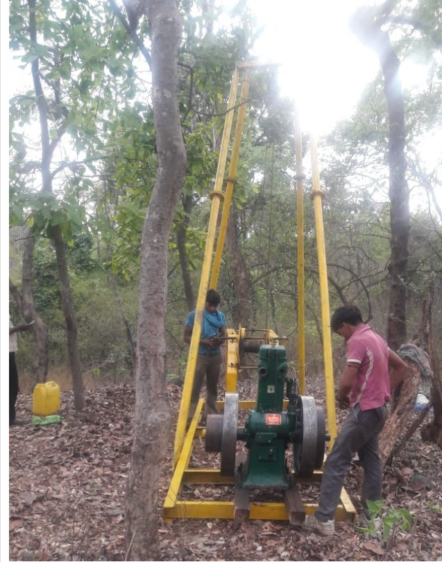
Bore Hole No. 5
