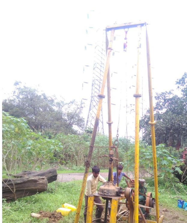
Bore Hole No. 1
