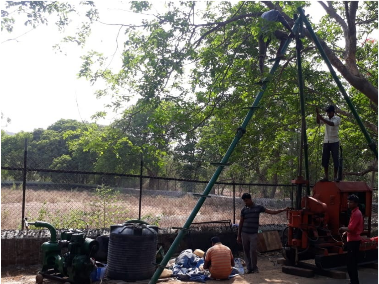
Bore Hole No. 8
