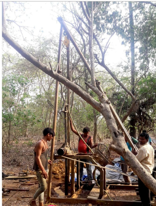
Bore Hole No. 4
