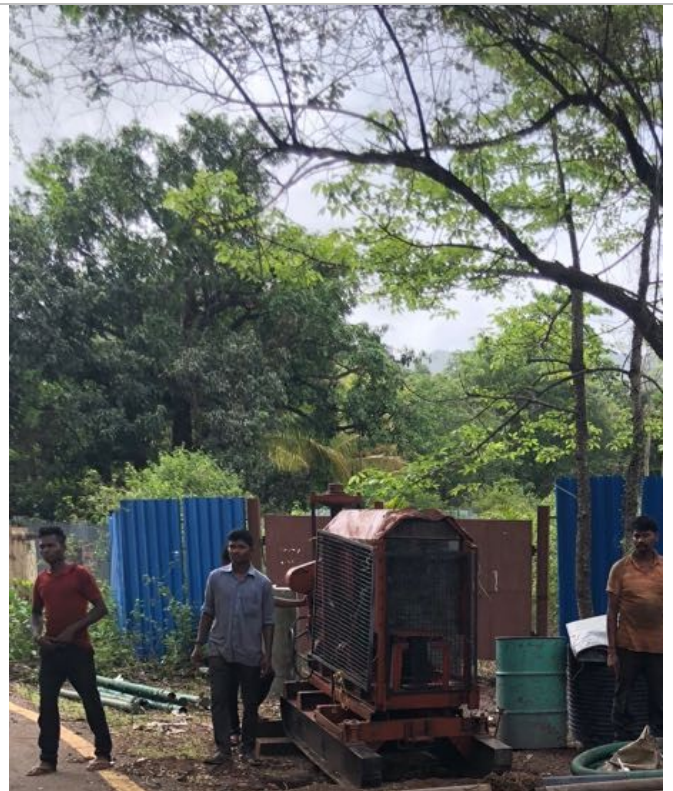
Bore Hole No. 9
